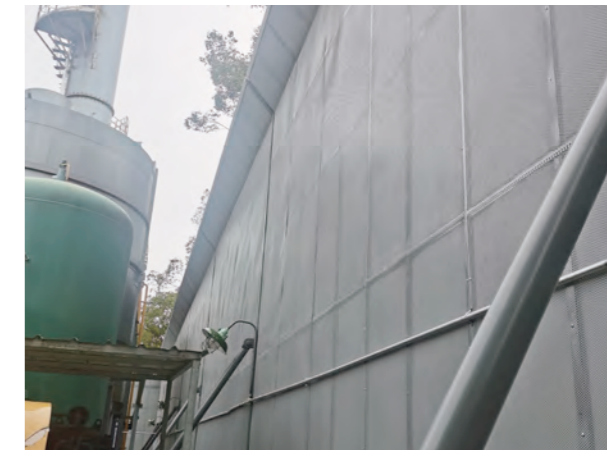
▲ 上海紫江彩印采用隔音墙保障作业人员职业健康。 Shanghai Zijiang Color Printing uses soundproof walls to ensure the occupational health of workers.
