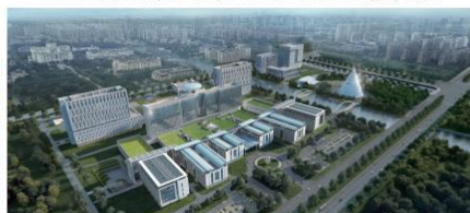
上海市第一人民医院南部院区二期扩建工程 Phase II Expansion Project of Shanghai 1st People's Hospital's Songjiang Campus
